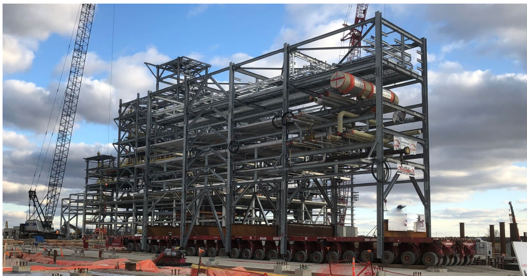
The first piperack module arriving to Rokeby Site.
