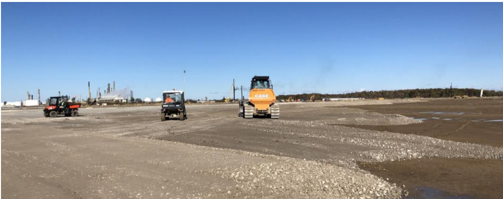
Parking lots and roadways are taking shape on the construction site.
