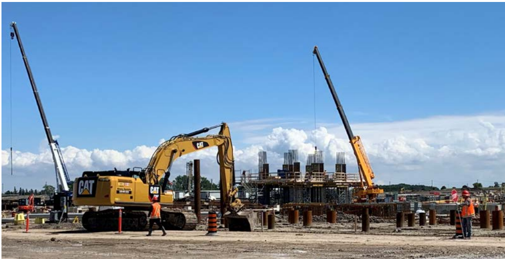
Foundations for the reactor structure rise from the ground.
