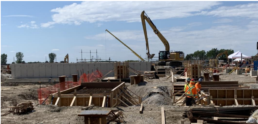
Rebar and foundation work continues in the Utilities area.
