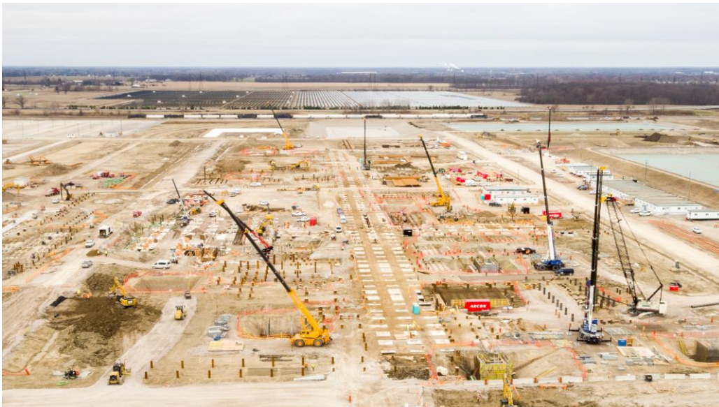
Aerial view of the construction site facing west.
