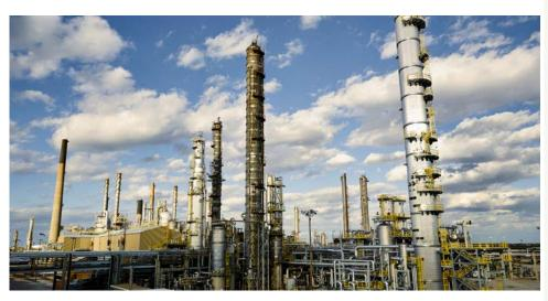
Feedstock Conversion: NOVA Chemicals converted its Corunna, Ontario manufacturing facility to use 100 percent natural gas liquids (NGLs), primarily ethane, as feedstock in 2010. The conversion has resulted in a 33 percent reduction in GHG emissions for our Ontario facilities; a 13 percent reduction for the company.
