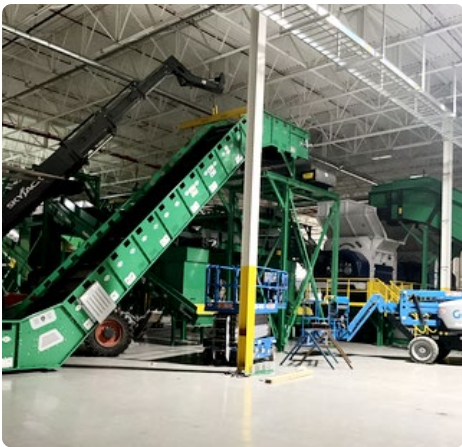
Sortation equipment is being installed and progressing as planned.
