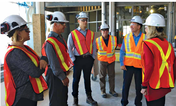
Our Leadership Team tours the construction site for the NOVA Chemicals Health & Research Centre at Lambton College — slated for opening next Spring.
