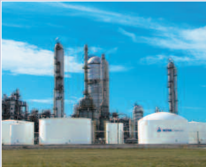
BAYPORT, TEXAS STYRENE MONOMER FACILITY
