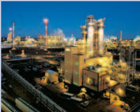
JOFFRE, ALBERTA, ETHYLENE/POLYETHYLENE FACILITY
