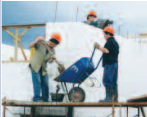
WORKERS BUILDING AN "ICF" HOUSE
