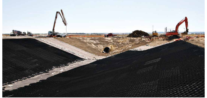
The new retention pond is expected to be complete this year.
