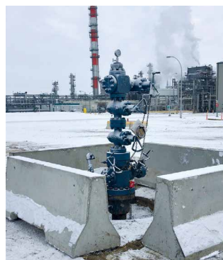
The new disposal well was drilled during the latter part of 2016 and completions work was done in January 2017.
